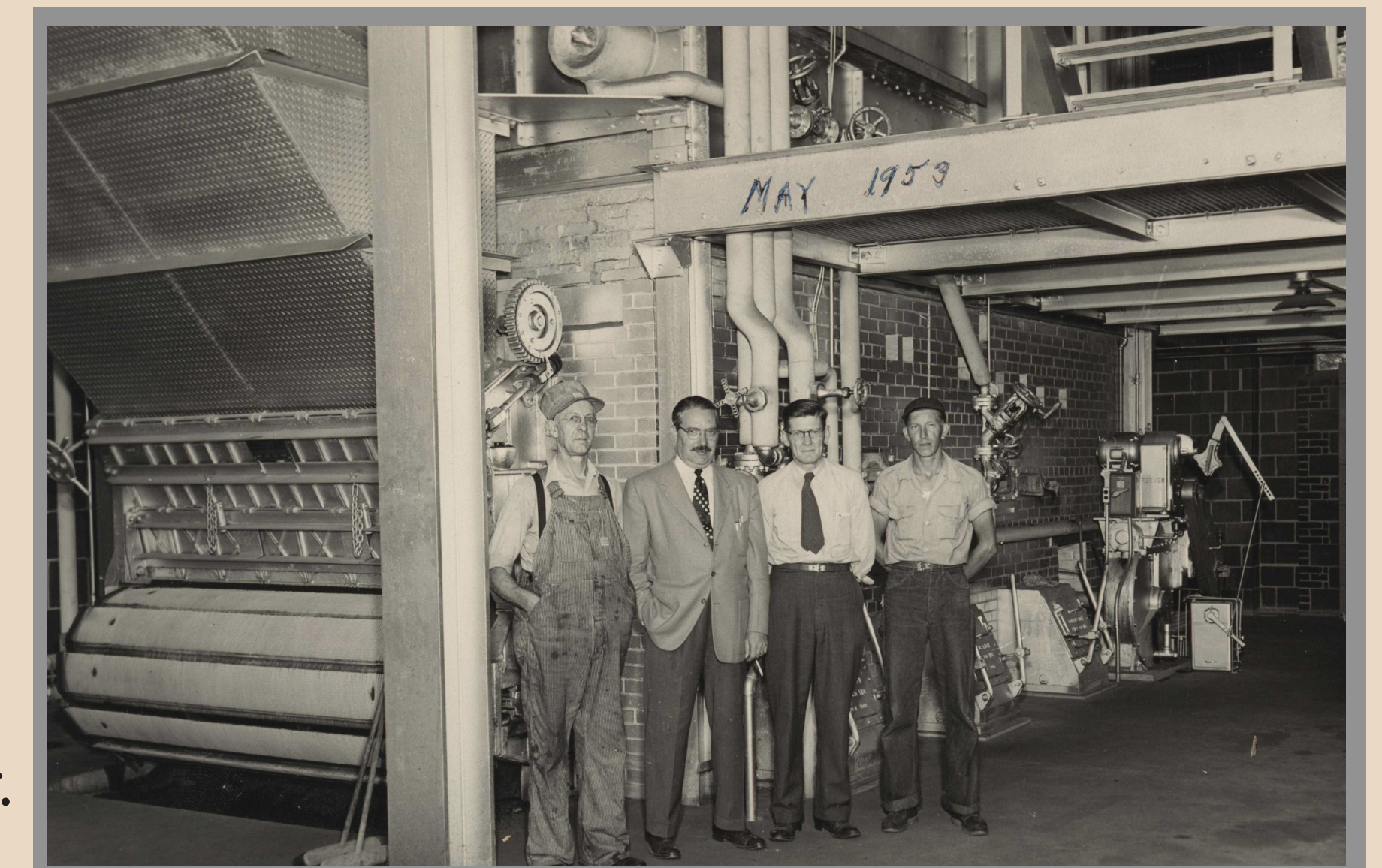
Interior of the Shippensburg State College steam plant, May 1953.
