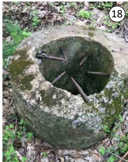
Electric pole base (Trindle Spring Segment)
